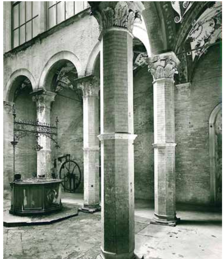
6b. Pilastrini ottagonali della corte interna. 6b. Octagonal pillars of the inner courtyard.
