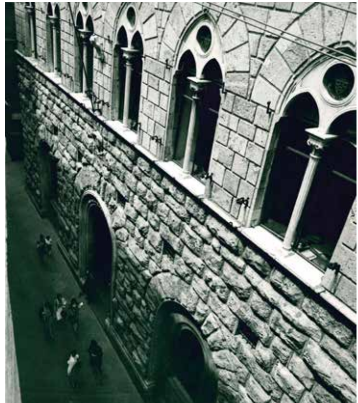
3b. Bifore a sesto acuto viste dall'alto. 3b. Pointed arch biforate windows seen from above.
